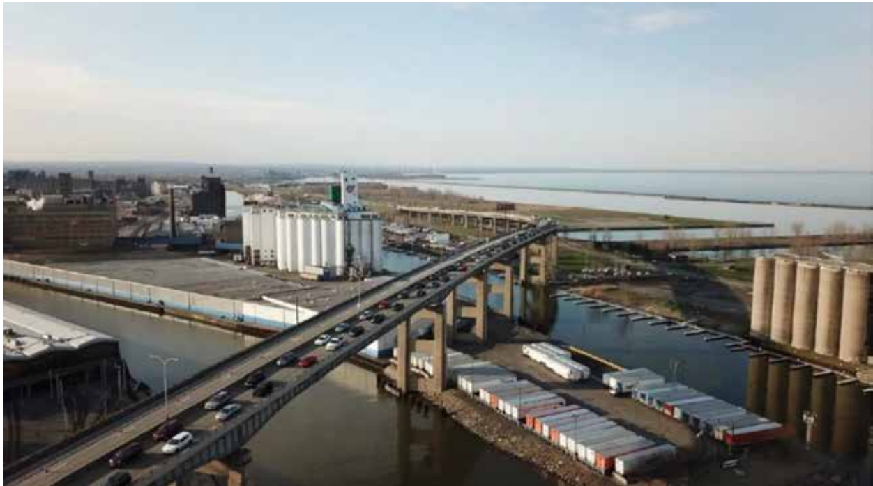
Fig. 3: Central portion of Skyway, crossing the Buffalo River and City Ship Canal, in foreground. The southern end of Skyway, Outer Harbor area, and Lake Erie are in background. John Hickey/ Buffalo News file photo; appeared in Buffalo News April 10, 2019.
