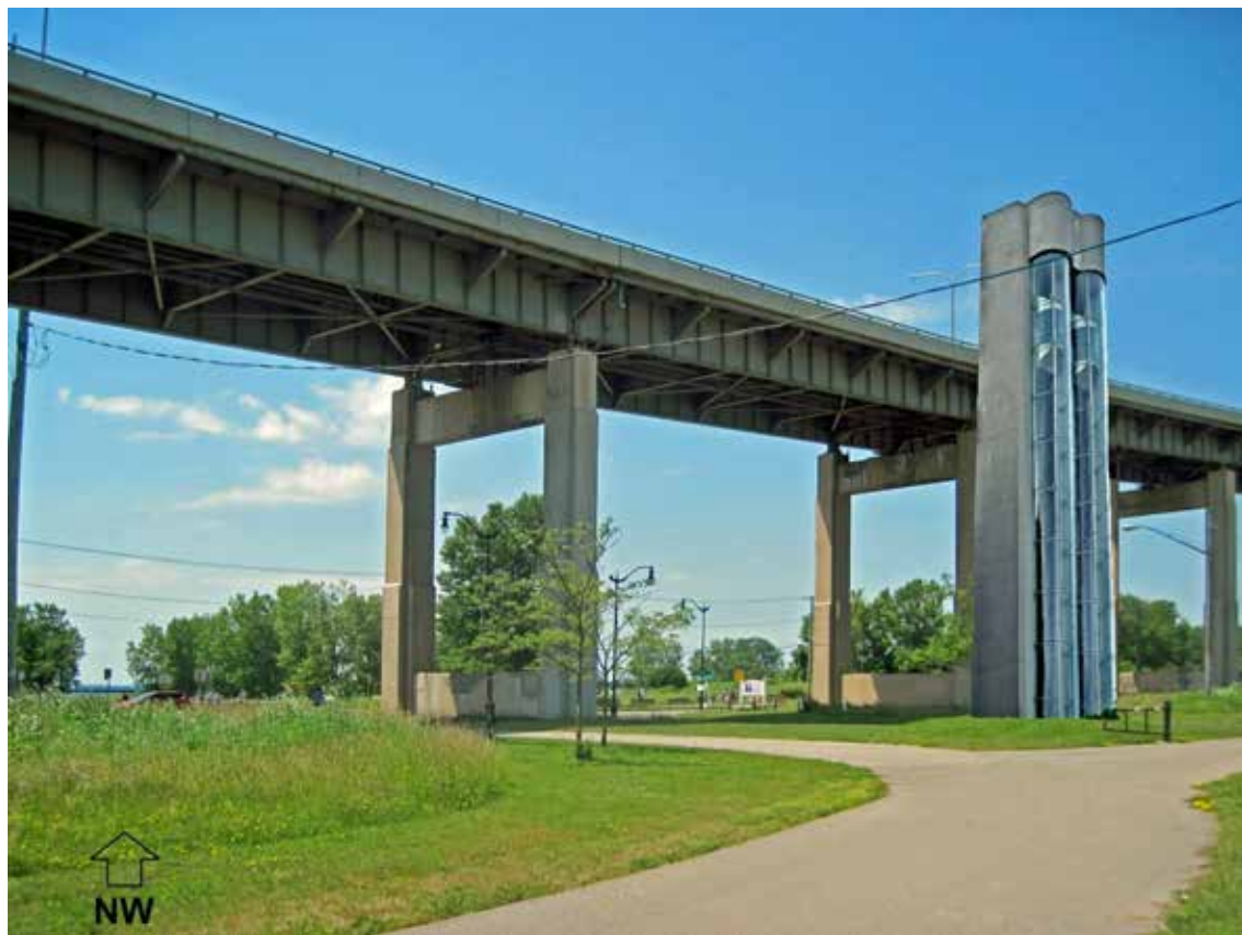
Fig. 10: Pair of elevators in the Outer Harbor near the intersection of Fuhrmann Blvd. and S. Michigan Ave., providing pedestrian and bicycle access to/from the repurposed Skyway. In combination with a similar pair of elevators at Canalside, the elevators pictured here will give pedestrians and cyclists a 2500-foot-long route across the Buffalo River and City Ship Canal via the Skyway. The elevator design shown here is based on the elevator at Marble Mountain, Da Nang, Vietnam.
